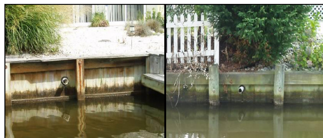
Figure 4. Examples of rooftop downspout and outdoor shower discharge directly into the Anchorage Canal
